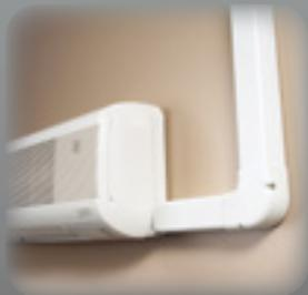
DiversiTech recommends attaching the base to the wall or ceiling and the line sets to the system every 15" to allow for the system to carry the full weight of the line sets.
