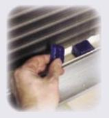
Place FLOW-PLUS<sup>TM</sup> in the condensate pan. FLOW-PLUS<sup>TM</sup> is a totally soluble long term polymer treatment that keeps the drain pan and condensate lines clean for a minimum of three months. This prevents pan overflow problems.
