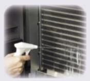
Disinfect and deodorize the evaporator coil and drain pan with SANI C-N-D<sup>TM</sup>, an EPA registered biocide, fungicide, viricide, and mildewstat. The broad spectrum biocide in SANI C-N-D<sup>TM</sup> assures control of many airborne pathogens that can be spread via contaminated air handling equipment.
