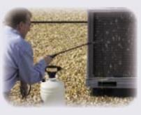
Clean the evaporator coil and condensate pan with TRIPLE "D"TM, a USDA authorized non-foaming alkaline coil cleaner. Cleaning the dirt from the coil and pan not only improves equipment efficiency, but also removes an important source of contamination that can create slime and sludge in the drain pan and cause pan overflow.
